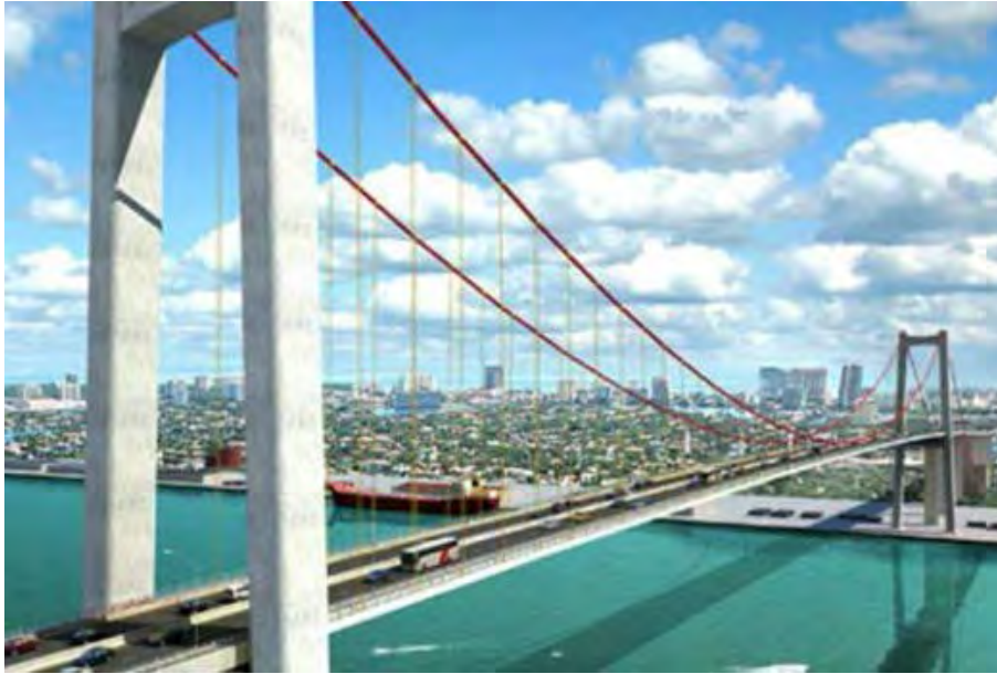
Bridge over Maputo Bay, Mozambique
