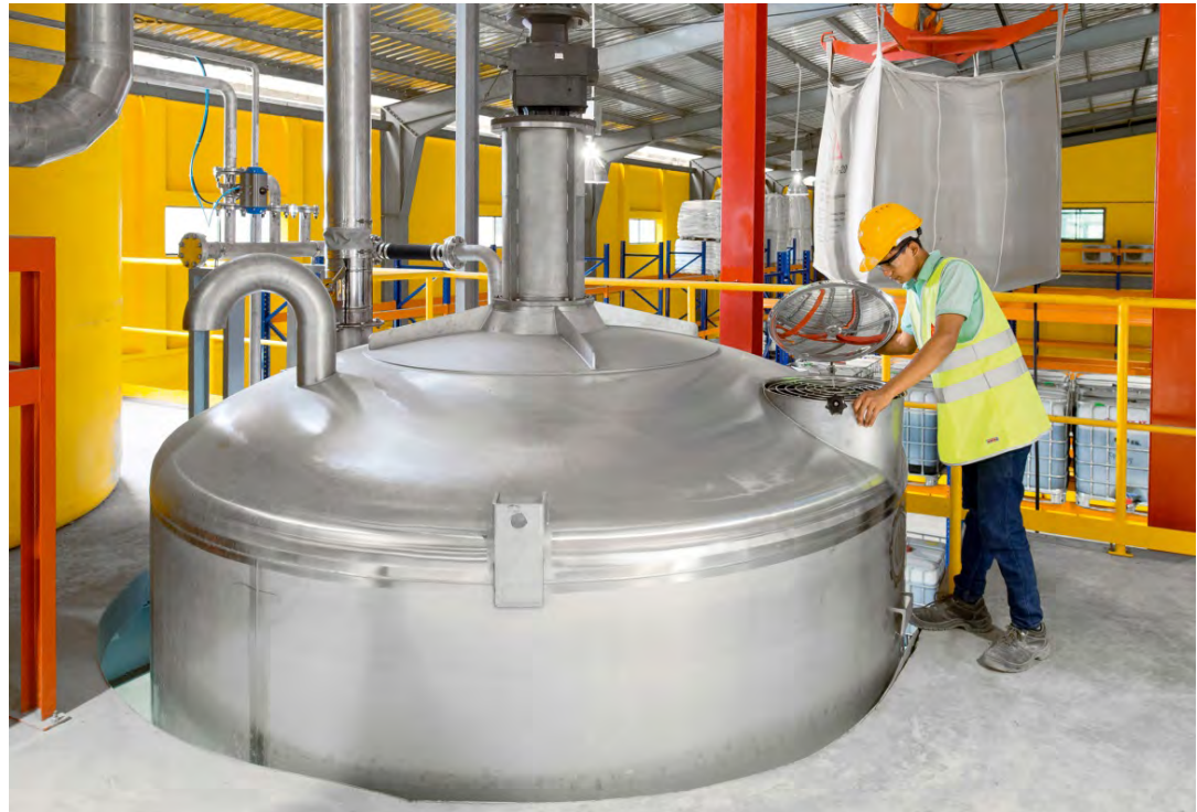
Sika Myanmar production facilities
